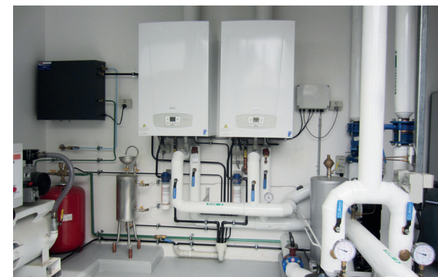
BAXI Duo-Tec MP+ condensing boilers in cascade w' APU, Hydraulic Separator
